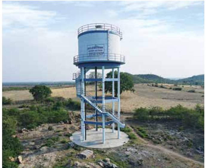
210 KL Overhead Service Reservoirs at Umara Village for Gadakota Multi Village Rural Water Supply Scheme in Sagar District in Madhya Pradesh.
