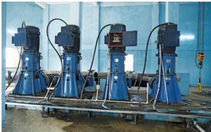
Installation of Pumping Machines of 75 KW (100 HP) Capacity VT Pump 4 nos at Bilaspur Water Supply Scheme in Chhattisgarh.
