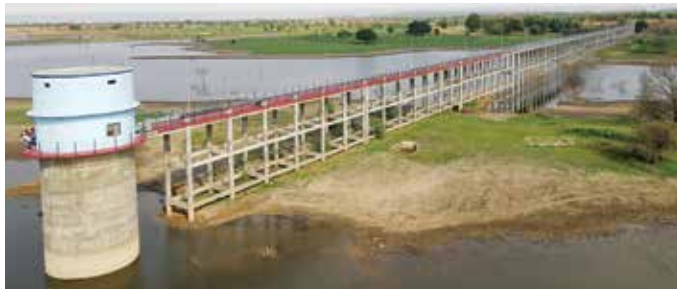
18.27 MLD of Intake Well cum pump house with Approach Bridge for a length of 630 meters for Gadakota Multi Village Rural Water Supply Scheme in Sagar District in Madhya Pradesh.
