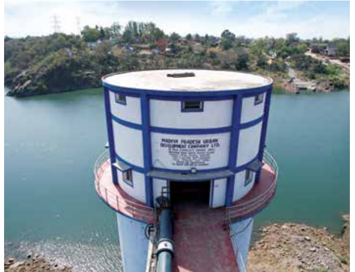
27.93 MLD Intake well cum pump house at Bhedaghat Town for Bhedaghat Water Supply Scheme in Madhya Pradesh.
