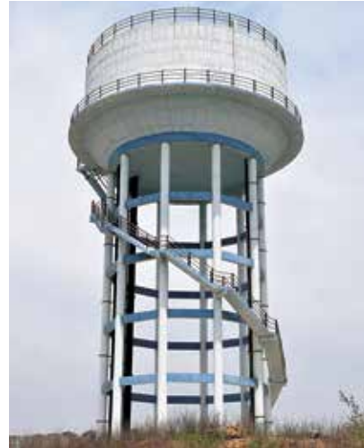
850 KL Overhead Service Reservoirs at Kandaila Multi Village Rural Water Supply Scheme in Rewa District in Madhya Pradesh.
