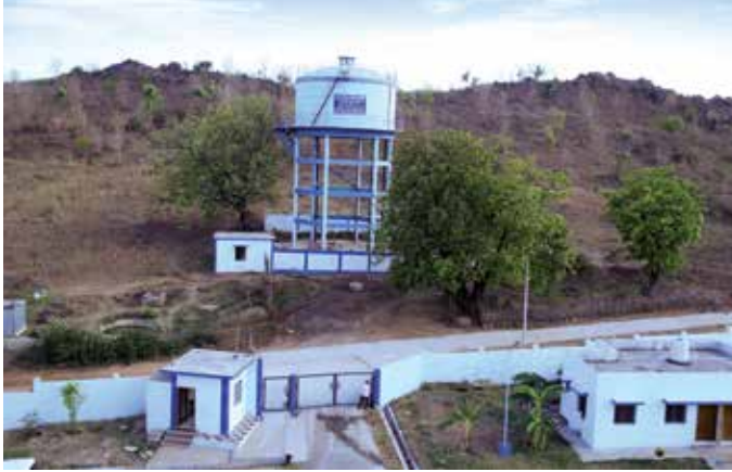
230 KL capacity Overhead tank at Jhal Village at Indwar Multivillage Rural Water Supply Scheme in Madhya Pradesh.
