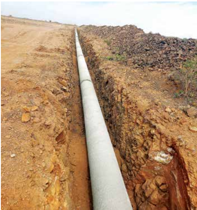
400 mm dia BWSC pipeline laying work at Man Canal PDN of Urmodi Irrigation Project in Maharashtra.
